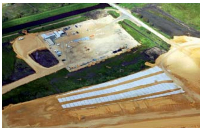
An aerial view of geofabric membrane laid at the Karnup Road interchange constructed as part of NPBH.
