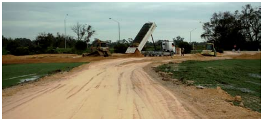
Construction underway at the Safety Bay Road interchange, Folly Rd, Baldivis
